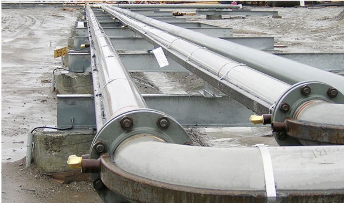
Application of Two ControTrace elements onto a Pipe
