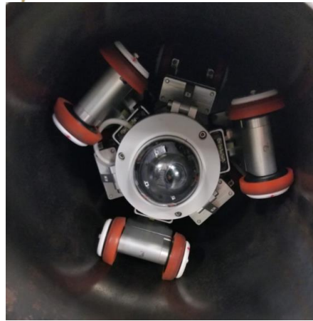
Figure 3: In-Pipe Visual Inspection
